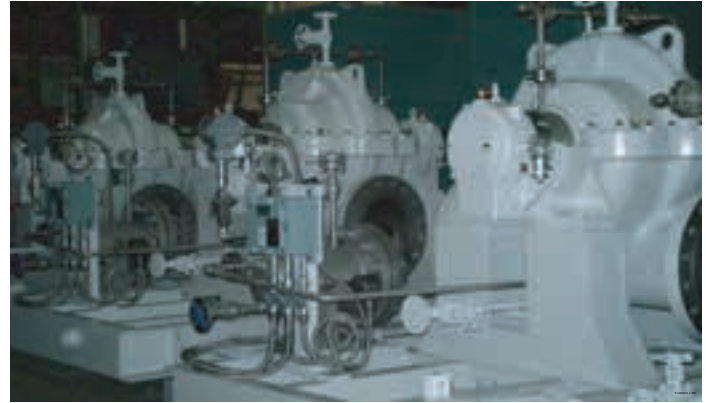
SPEC : 1100 m 3 /hr x 93 m x 350 kW x 1485rpm
